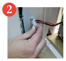
2-Open the plastic clamper to take out the cables
