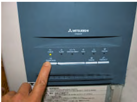
Turn on the power, then press the Door Open button.
