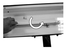
Carefully twist the lamp to remove.
